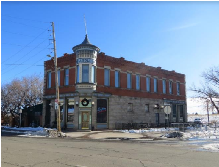
The J. Solf Building at 2644 West Colfax Avenue. Discover Denver photograph.
