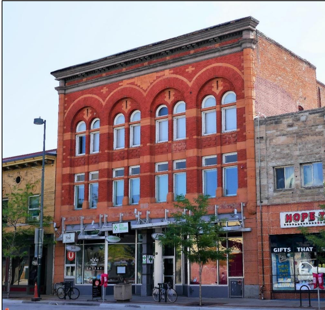
The Fleming Brothers Building, constructed in 1890. Discover Denver file photograph, July 12, 2018.
