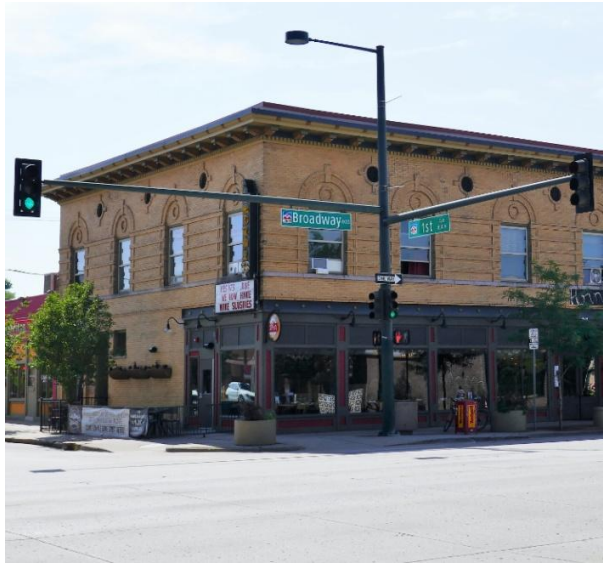
76 N. Broadway, constructed c.1900
