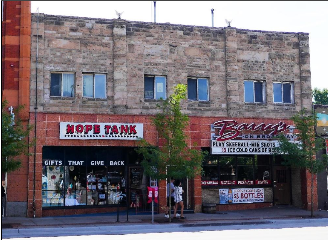
58-64 Broadway, constructed 1913. Note the visible lintels in the upper wall, indicating the original window height. Discover Denver file photograph, July 12, 2018.
