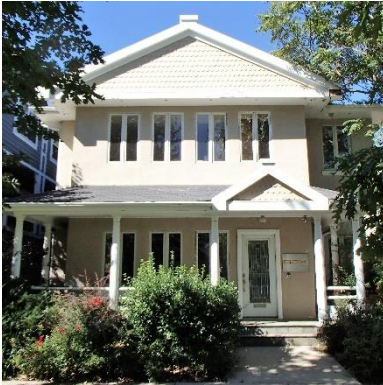
1761 Emerson Street, constructed 1902. Alterations include a dominant second-story addition and complete window and cladding replacement.
