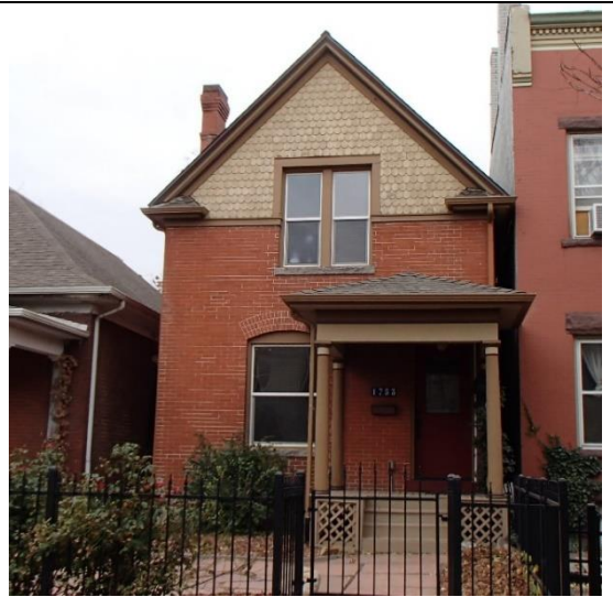
1759 Washington Street, constructed 1906
