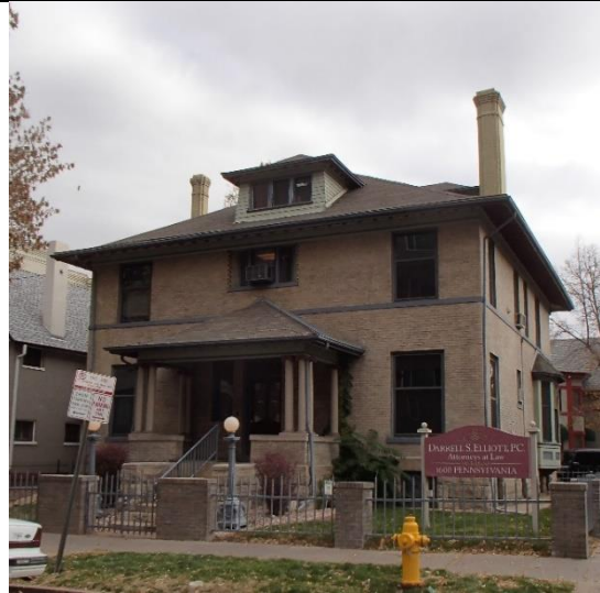
1600 Pennsylvania Street, construction date unknown (prior to 1929).
