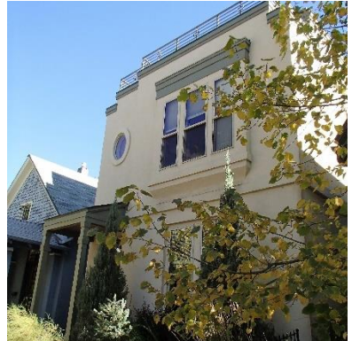
1722 Washington Street, constructed 1890. Alterations include modern stucco siding, window replacements, and rooftop deck railing.
