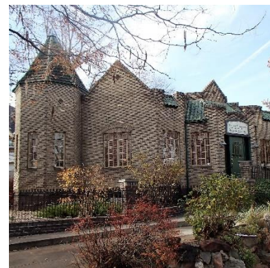
1717 Downing Street, constructed 1940.
