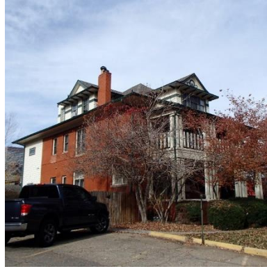
1647 Clarkson Street, constructed 1906. Alterations include a 2-story rear addition.
