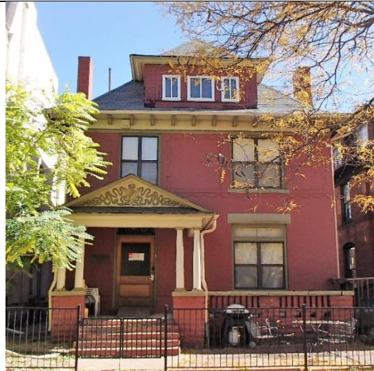
1616 Washington Street, constructed 1896
