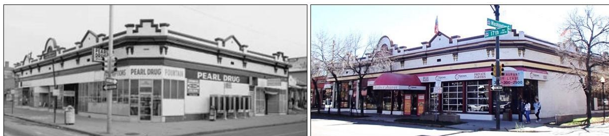
700 E. 17 th Avenue, a one-part commercial block building that housed Cliff Young’s and other historically significant establishments. Shown at left in 1981 and at right in 2017. Sources: Denver Public Library Call no. No. Z-10446, http://digital.denverlibrary.org/cdm/ref/collection/p15330coll22/id/83104 ; Discover Denver file photograph, October 21, 2017.
