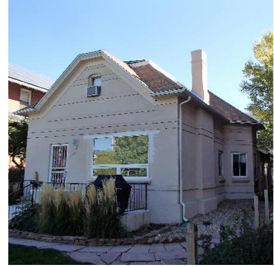
1738 Emerson Street, constructed 1920. Alterations include porch removal and window enlargement.
