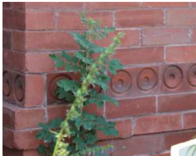
Decorative pressed brick found on all seven houses in J. F. Howell's Subdivision.
