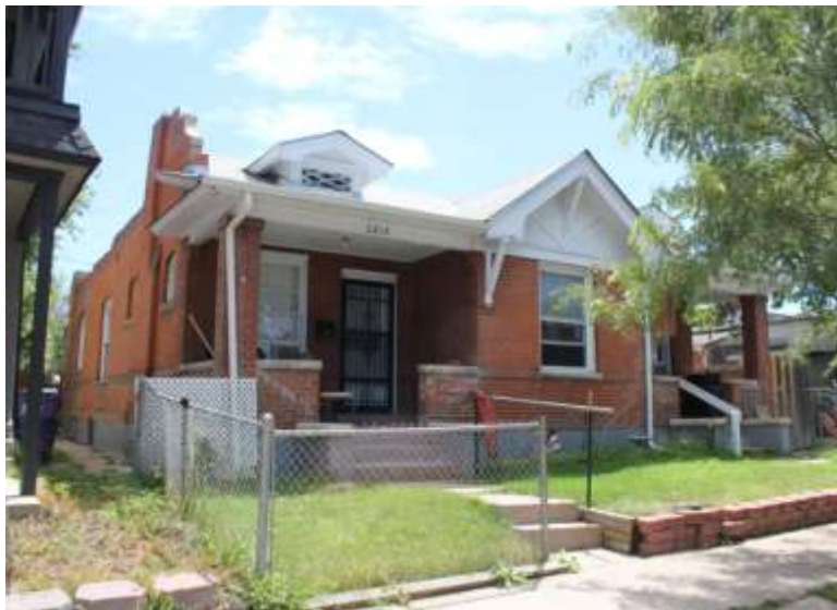
2814-2818 Eliot Street: One of several Craftsman-style duplexes in the Northwest Jefferson Park area.
