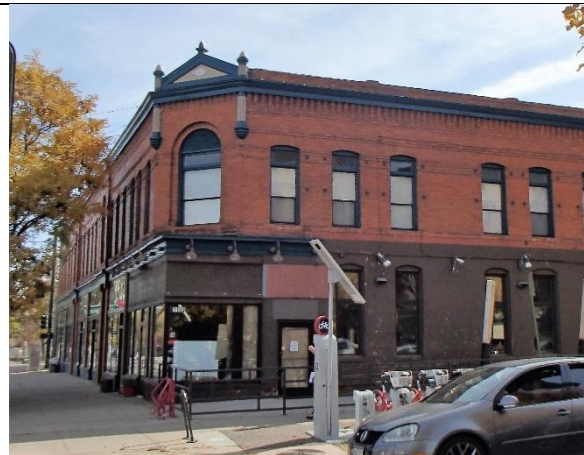
Italianate style building. Upper floor is chamfered but lower floor is built out. 1100 E. 17 th Avenue, Baerresen Brothers, architects, constructed 1890.
