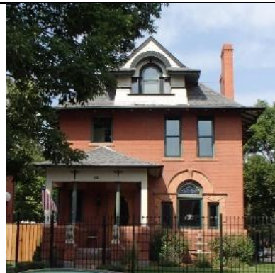
Early example with asymmetrical upper façade. 2155 N. High Street, constructed 1894
