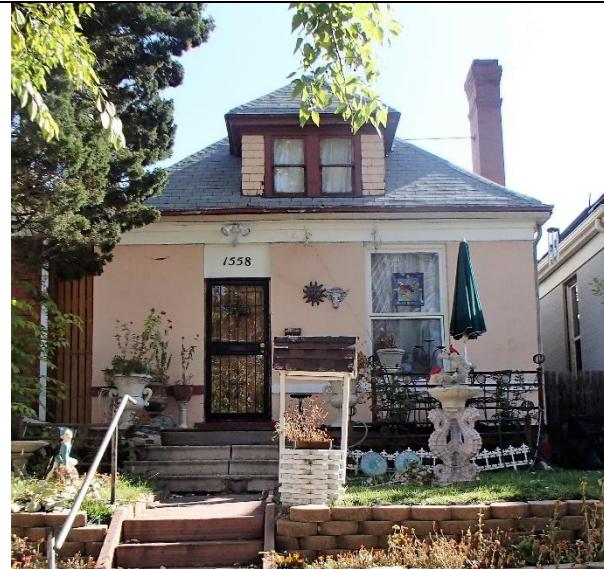
An early example of the Classic Cottage form, this house has no eaves and no covered porch. 1558 Marion Street, constructed 1893
