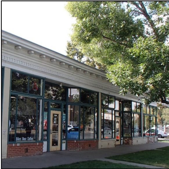
A row of storefronts facing north on E. 17 th Avenue at Lafayette Street.
