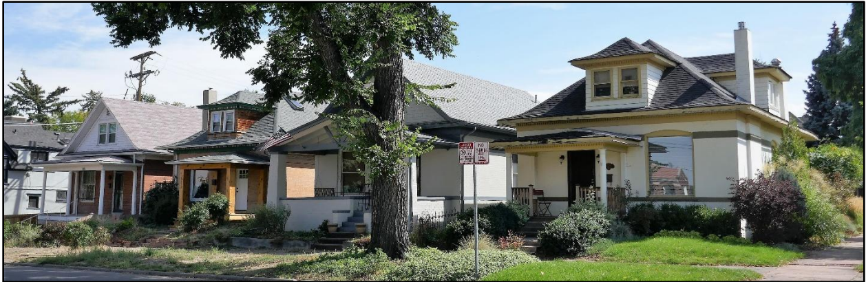
This row of four Classic and Victorian cottages at E. 23 rd and Gaylord was built in 1898 and designed by architect Charles Quayle.
