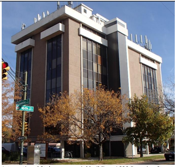
International Style commercial building, 1600 Downing Street, constructed 1973.
