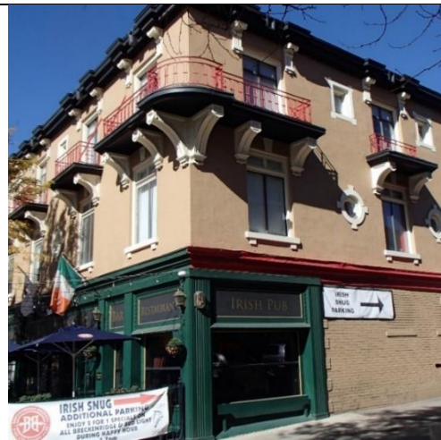
Former hotel with Italianate and Classical Revival elements. 1201 E. Colfax Avenue, constructed prior to 1929
