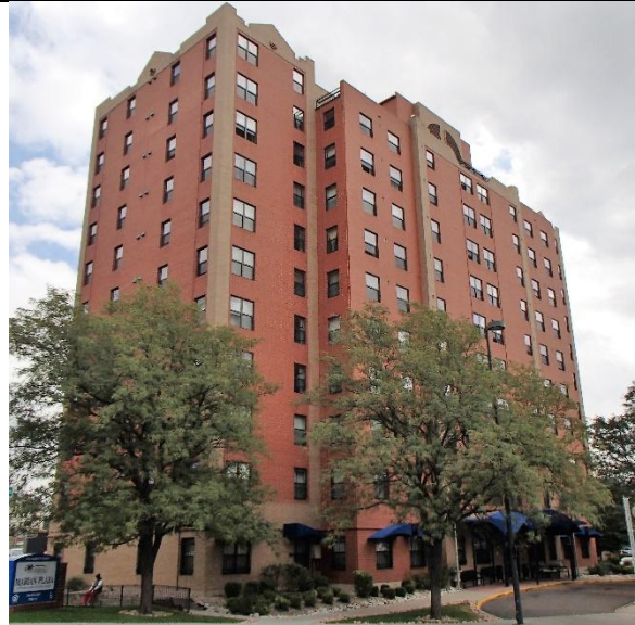
Postmodern style evident in the shaped parapet. 1818 Marion Street, constructed 1982
