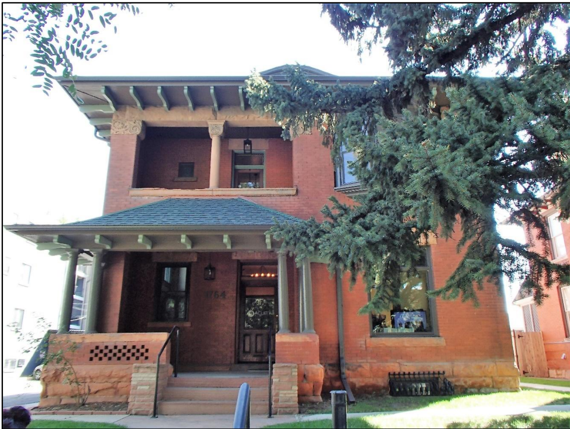
1764 Gilpin Street, 1892. James Murdock, architect. Discover Denver file photograph.
