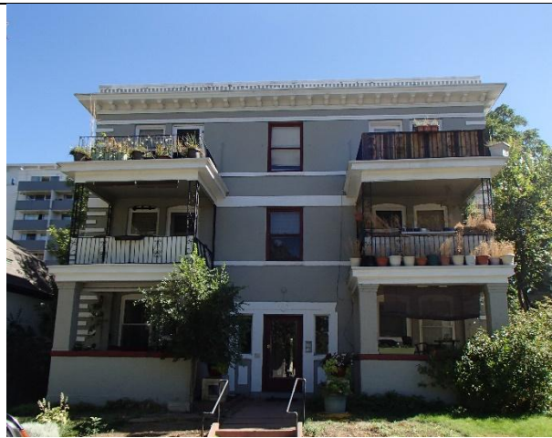
Stacked balconies on front façade, with interior entrance at center. 1560 Gilpin Street, constructed 1904
