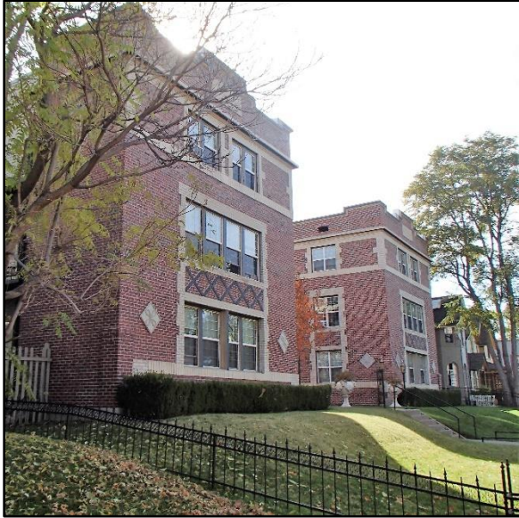
The Kenilworth Court Apartments, 1560 Downing Street, constructed 1908.
