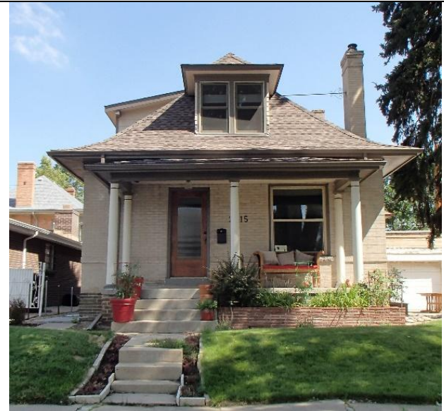
Typical Classic Cottage with Classical Revival porch columns, 2015 E. 21 st Avenue, constructed 1905 (left side shed dormer is a recent alteration).
