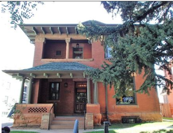
Early example of the Foursquare form with late Victorian elements. 1764 Gilpin Street, James Murdock, architect, constructed 1892
