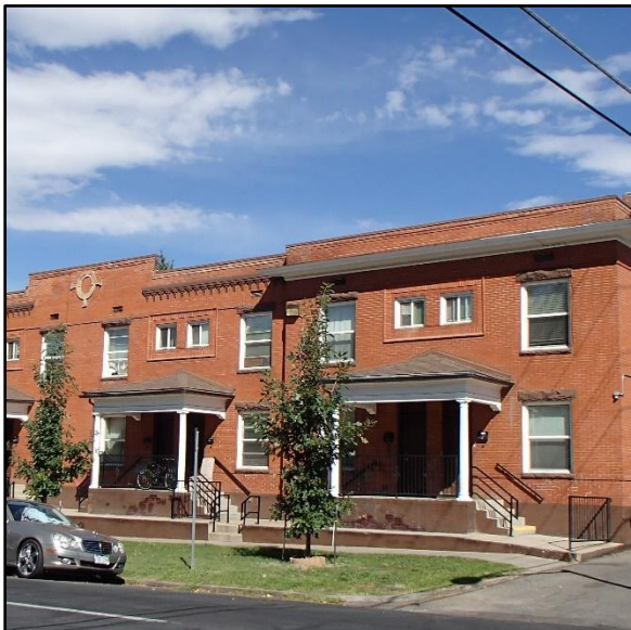
Rowhouses at 1601 E. 17 th Avenue designed by architect John Huddart and constructed in 1902.
