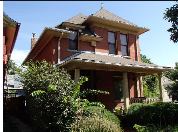
Early Edwardian style, 1639 E. 22 nd Avenue, constructed 1898
