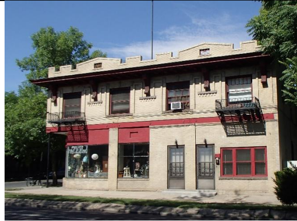
Renaissance Revival style building with chamfered corner entrance. 2219-2225 E. 21 st Avenue, constructed 1920.
