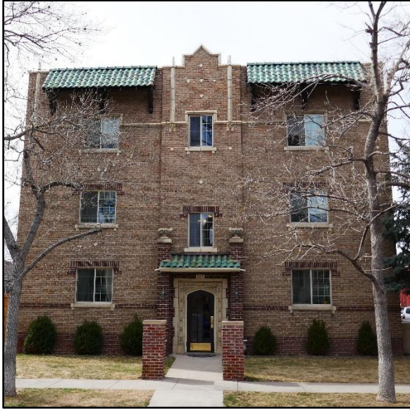
967 Marion Street, constructed 1929
