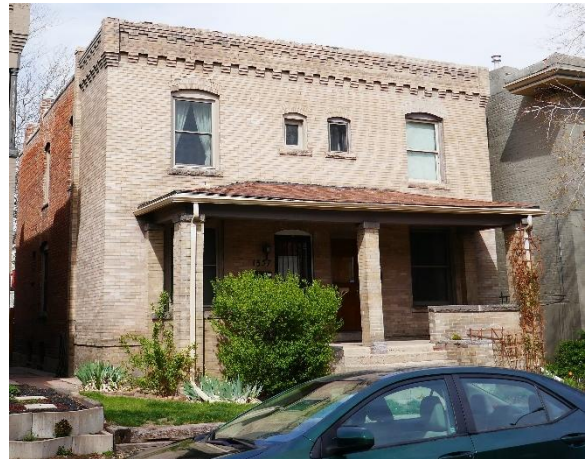
1357-59 Marion Street, constructed 1901
