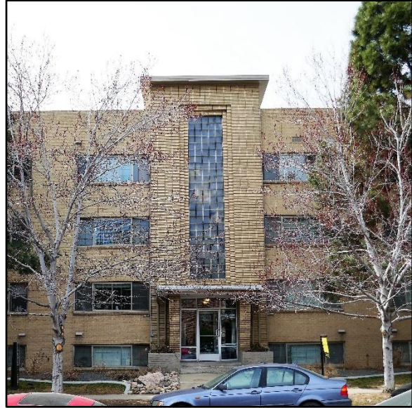
929 Marion Street, constructed 1955
