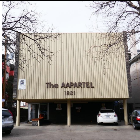
1221 Clarkson Street, constructed 1962
